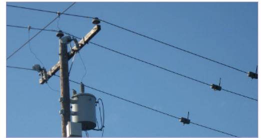
*A Wireless powerline sensor hangs from an overhead power line and sends measurements to a data collection system. Overhead power line monitoring helps distribution system operators provide reliable service at optimised cost.*
